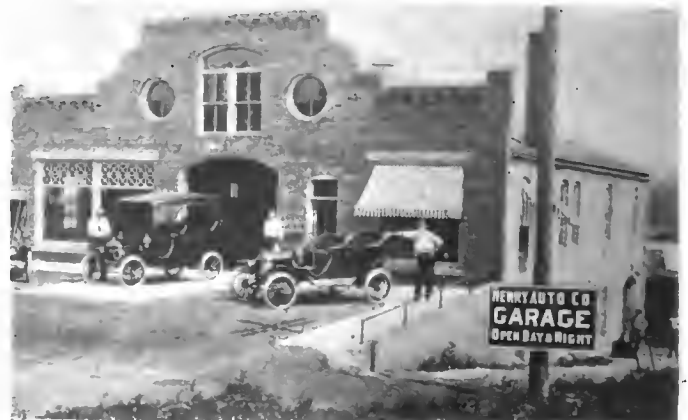
Henry Garage, with second floor down stairs.
